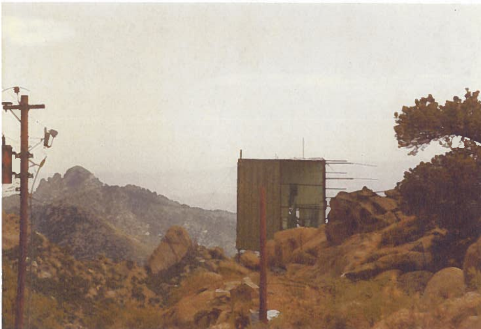
C5 houses backup to translator antennas in a stacked configuration.
