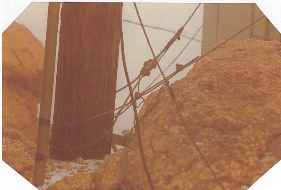
Antenna guy connects on top of peak.
